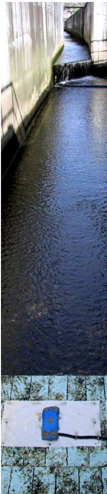
ADFM Pro20 Installation
