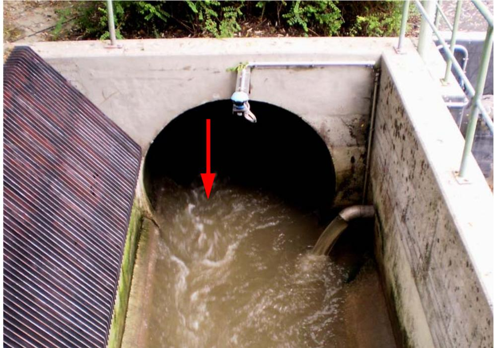
**Figure 1: WWTP inlet channel** Peak velocities visible on left side of pipe (red arrow).
