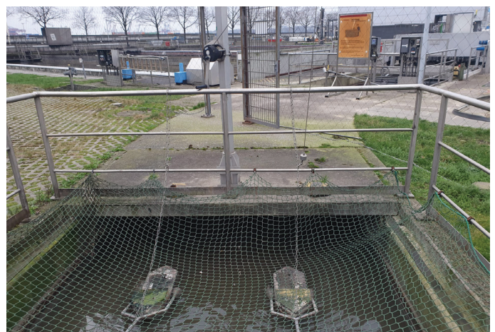
Existing contact sensors attached to floats at inlet channel of Köhlbrandhöft WWTP.
