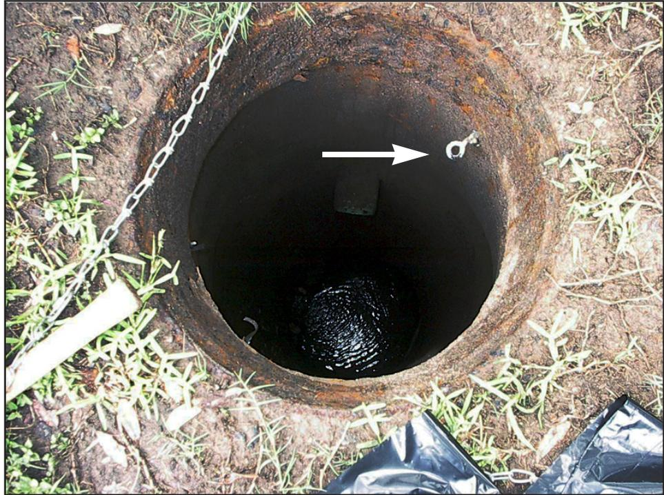
Figure 2-24 Lag shield - eyebolt manhole mounting
