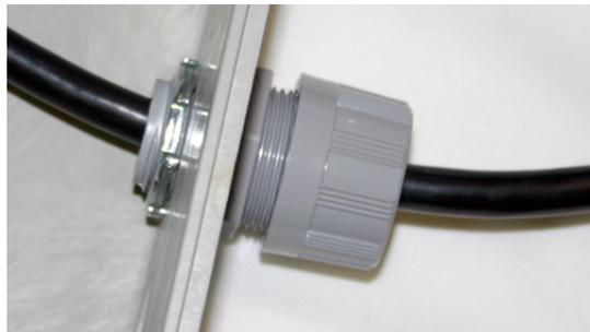
Figure 2-10 Position and secure the cable
