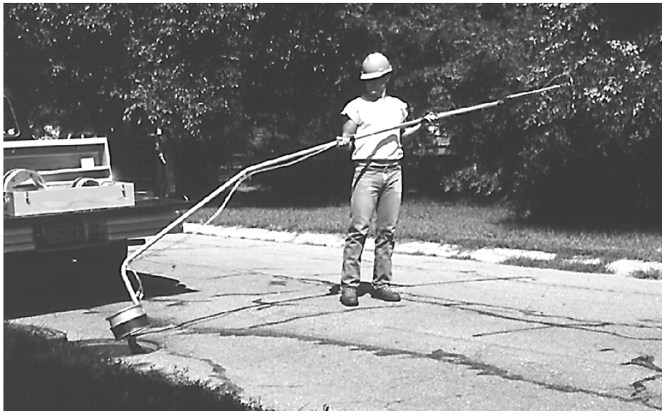
Figure 3-7 Lowering the Flow Poke into the Manhole
