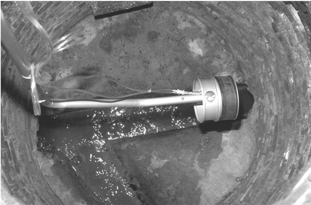
*Figure 2-8 Insert Lowered to Bottom of Manhole*
