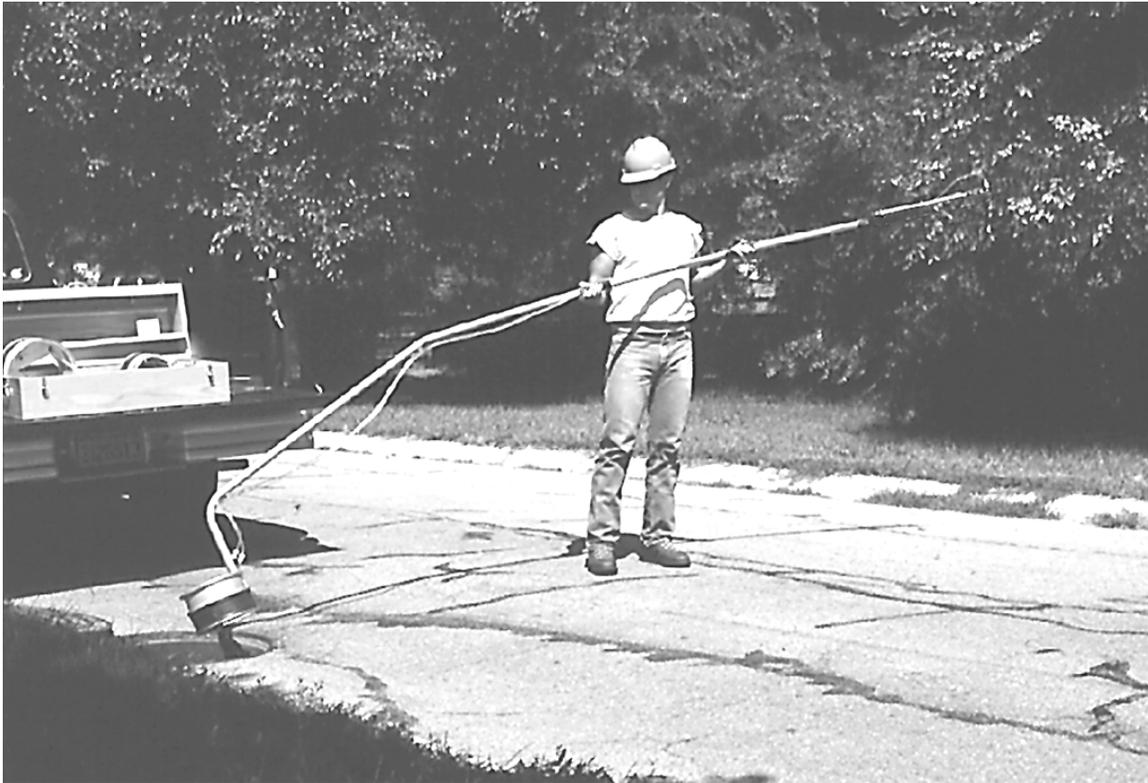
*Figure 2-7 Lowering the Insert Into the Manhole*
