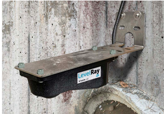
Figure 2-1 Wall mount with the LevelRay sensor installed
