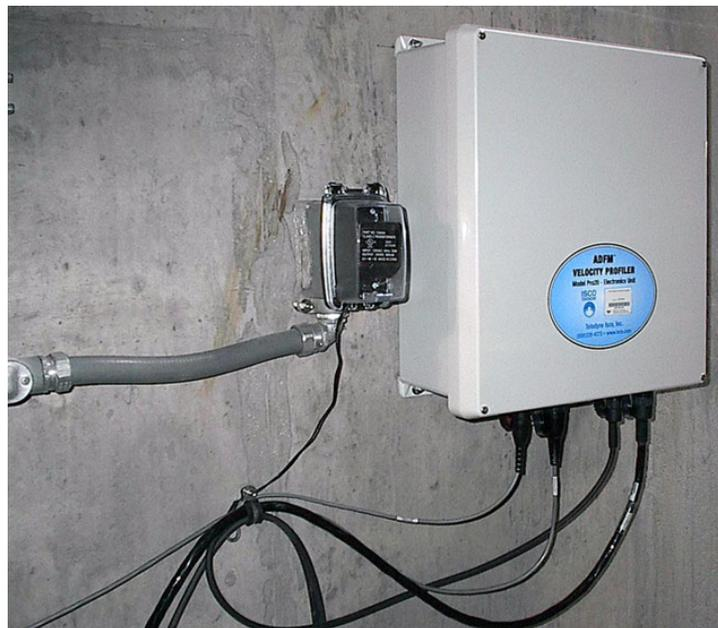
*Figure 2-19 ADFM controller: wall mounting*
