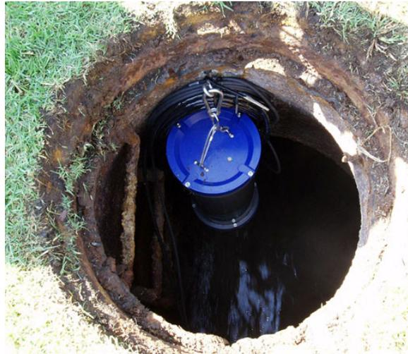
Figure 2-21 ADFM controller: cylindrical canister suspended in manhole
