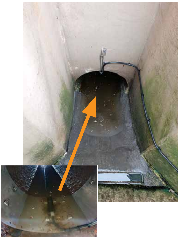
A 350 Ex AV sensor installed in an overflow channel using a mounting ring.
