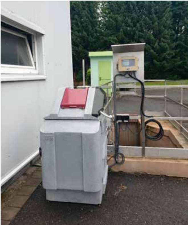
A Teledyne ISCO 5800 sampler and Signature flow meter installed at Kelč wastewater treatment plant.
