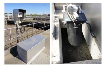
Figure 1: Signature flow meter with LaserFlow sensor sheltered in weather encloser
