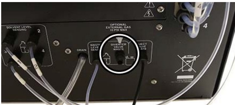
Figure 3-25 Diverter Valve Waste port with no connection
