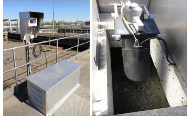
Figure 1: Signature flow meter with LaserFlow sensor sheltered in weather enclosure
