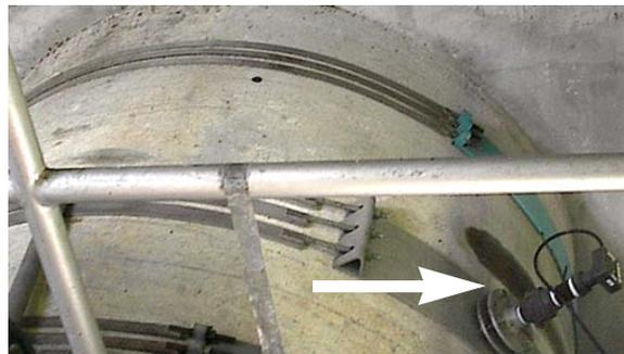
**Hot Tap sensor installed in pipe**
