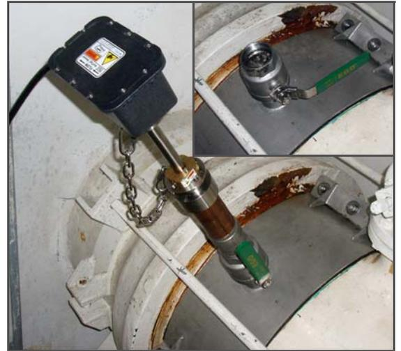
**Figure 2: ADFM Hot Tap sensor installation**
