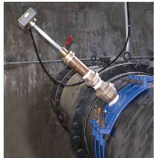
The ADFM Hot Tap sensor installs through a standard two-inch tap.
