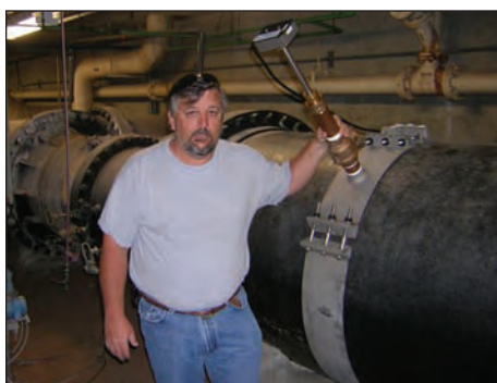
Lester Hendrix with Hot Tap installation
