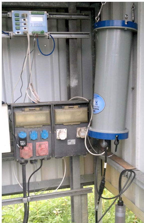
ADFM Pro20 canister electronics unit (IP68) installed with accQcomm Interface Module
