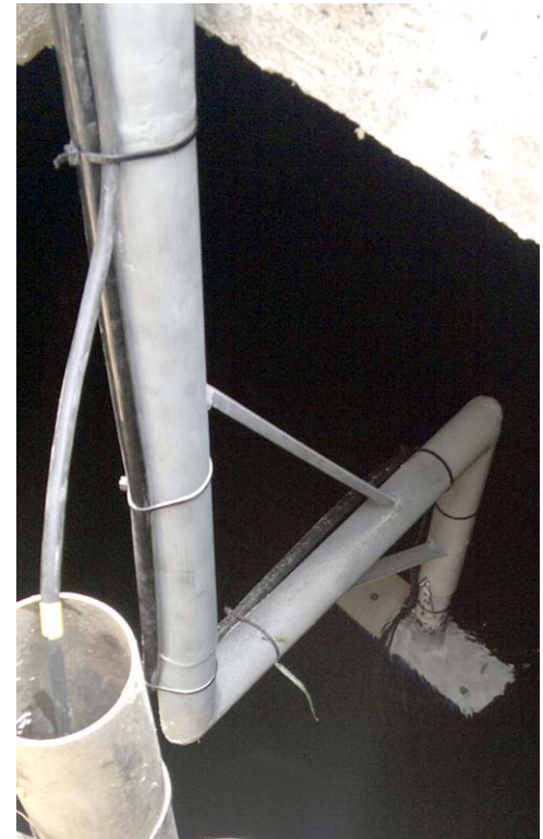
ADFM Pro20 sensor top mounted in a cooling water channel (red arrow)
