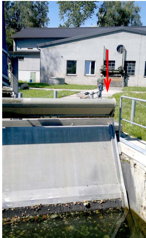
ADFM Pro20 sensor top mounted in a cooling water channel (red arrow)
